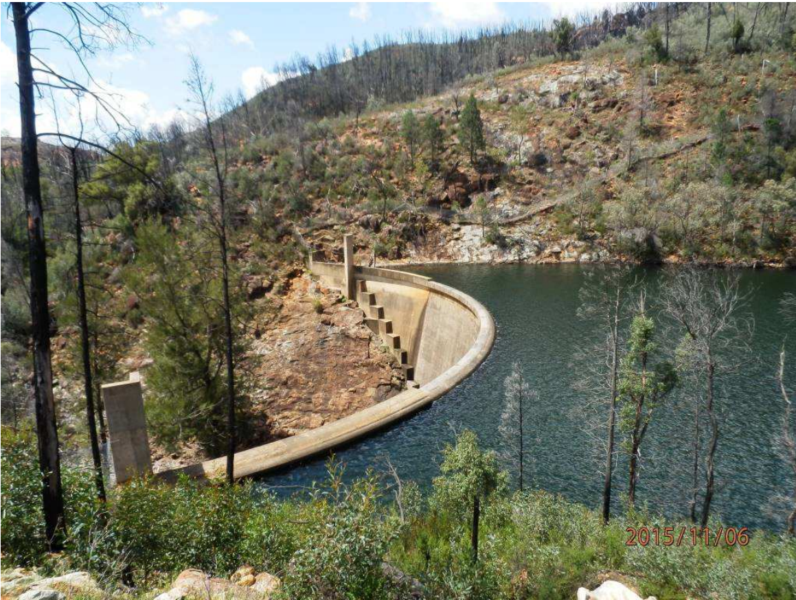
Photo 1: General view of the dam from left hand side
