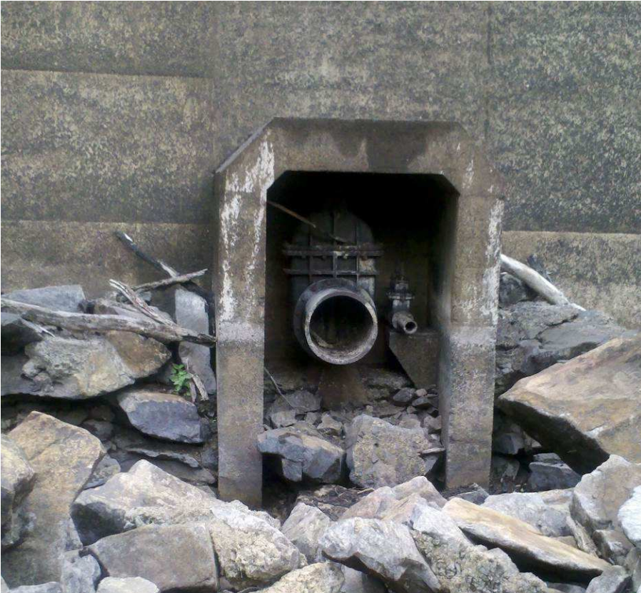
Photo 10: Scour Outlet (photo taken by council staff in June 2014)
