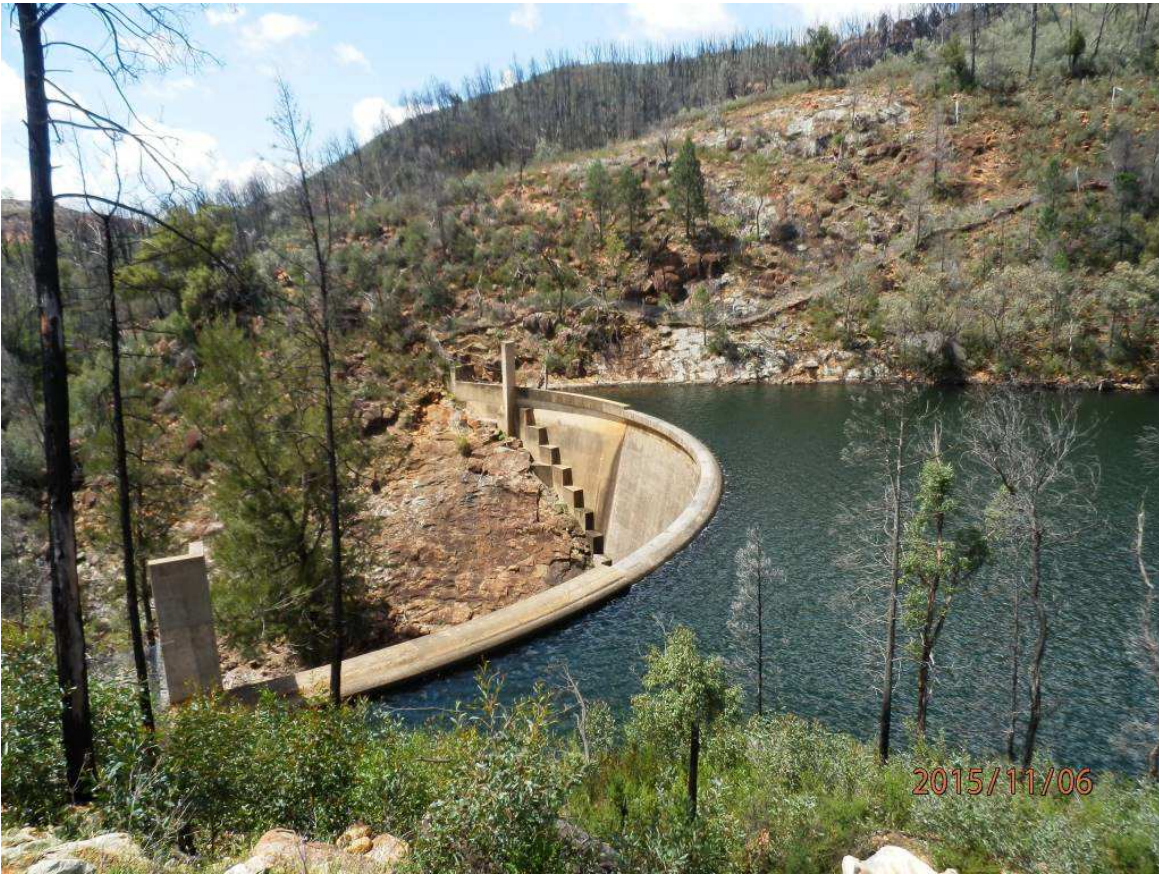
Photo 5: Dam crest (and unsubmerged portion of upstream face)
