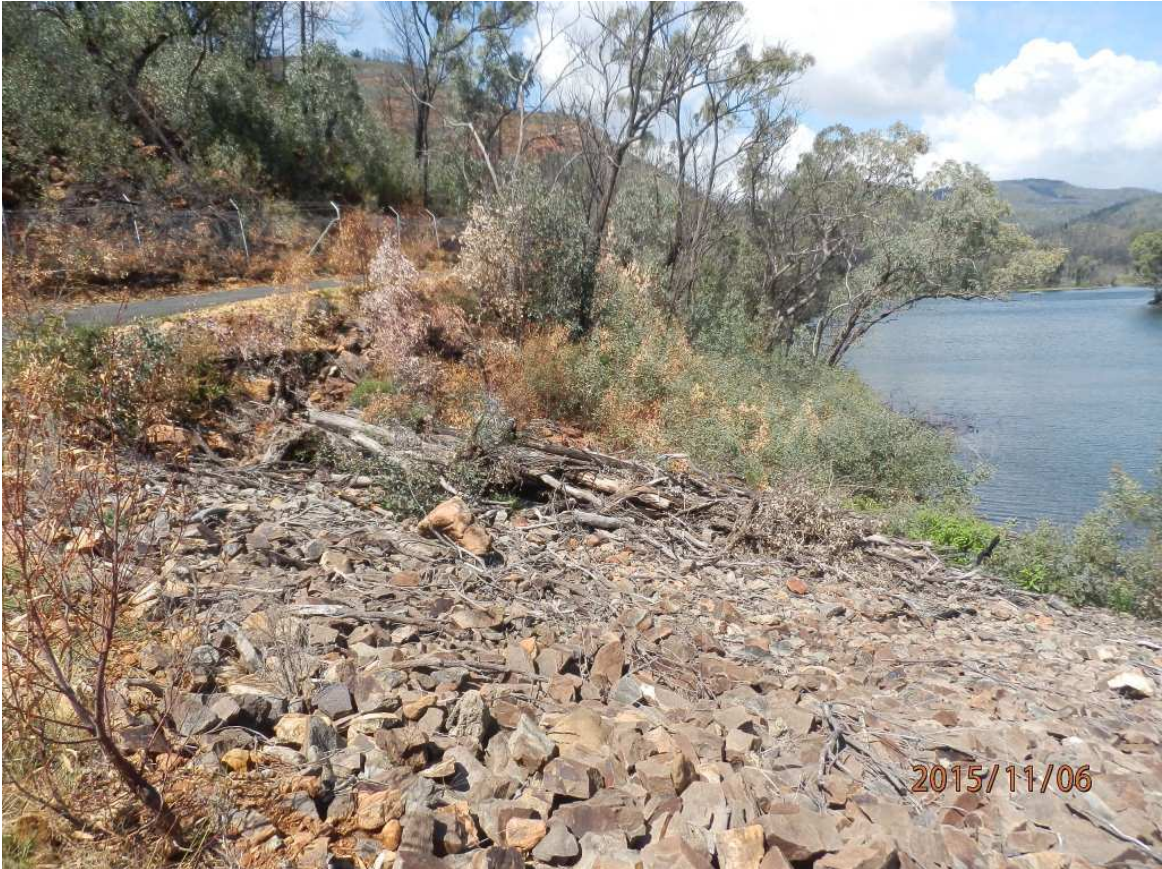
Photo 14: Saddle dam right abutment upstream side
