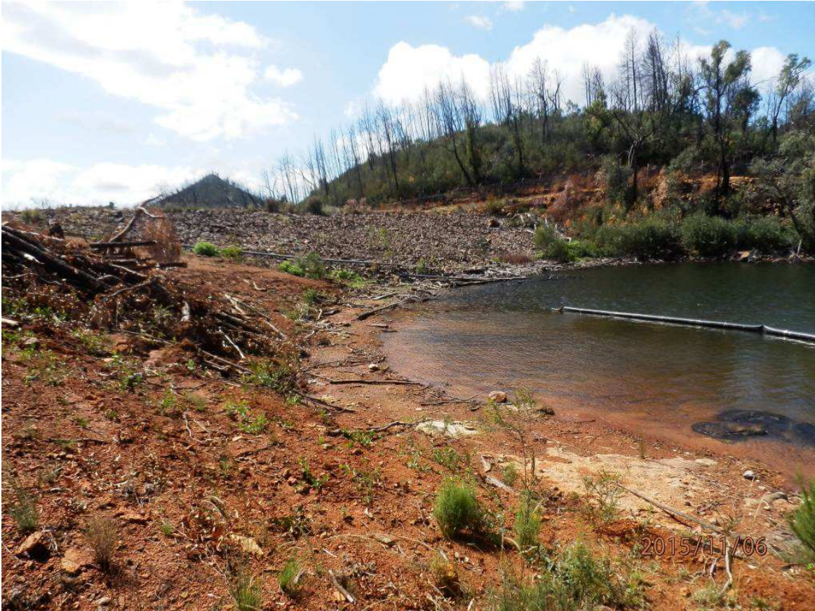
Photo 13: Saddle dam upstream face
