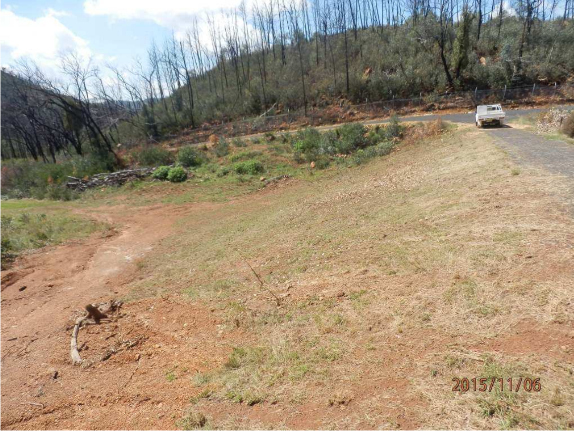
Photo 12: Saddle Dam downstream face
